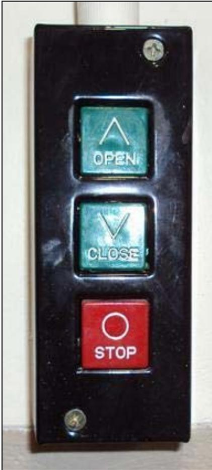
UWM Univ. Services and Research Building, March 2012: positive control switch for a new overhead door (close action will cease if button is depressed). Some older doors have the same style switch which are not positive control; in other words the door will continue to close if the switch is depressed.
